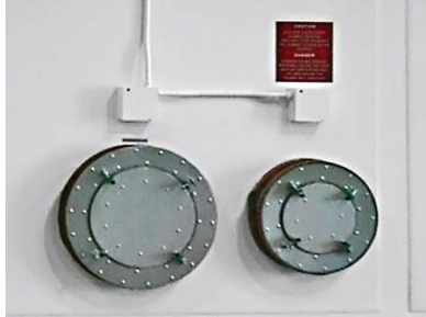
Access ports furnished with a flexible diaphragm to compensate for inner liner movement at -180 C.
